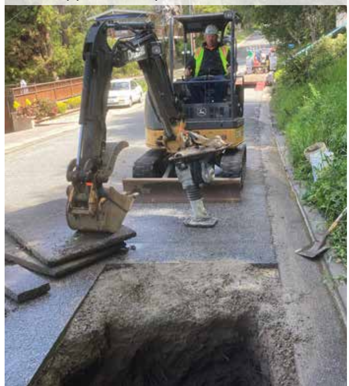
In 2021, 15 water main pipeline leaks and 90 service pipelines were repaired.
