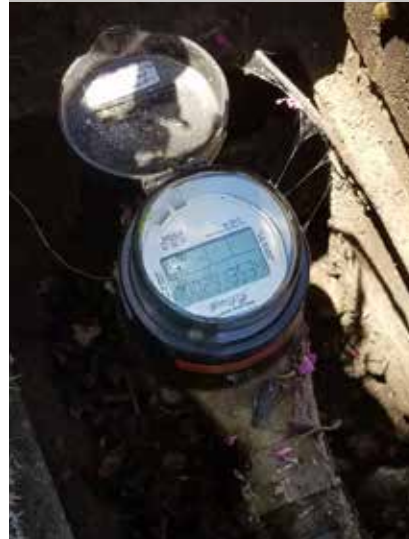
District water meters are now upgraded to i-Meters (intelligent-metering technology), making it easier for customers to track water use and receive leak alerts.
