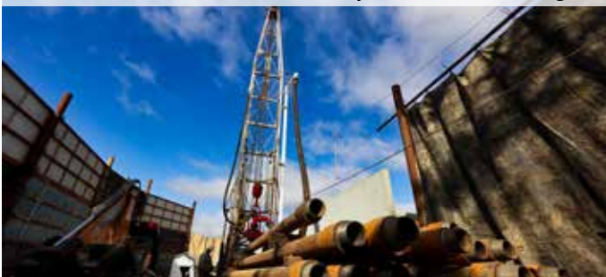
Willowbrook Lane seawater intrusion prevention well drilling.
