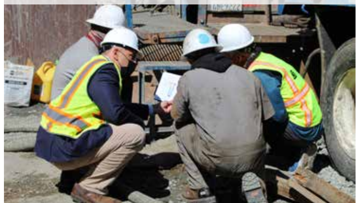
Congressman Panetta visiting a seawater intrusion prevention well construction site.
