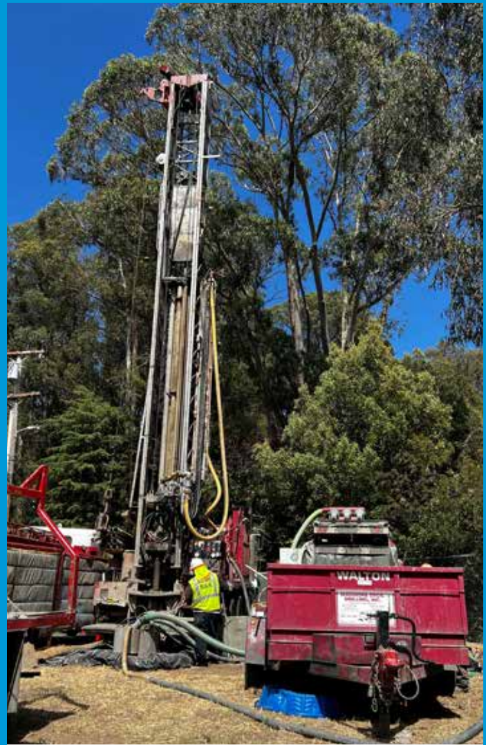
The MGA built an additional monitoring well in the Capitola area to obtain a better understanding of seawater intrusion.
